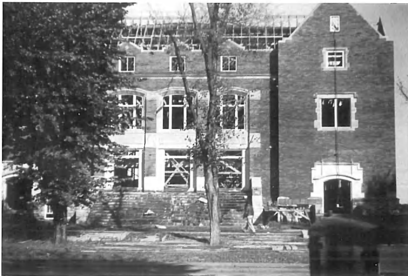
Memorial Hall under construction
