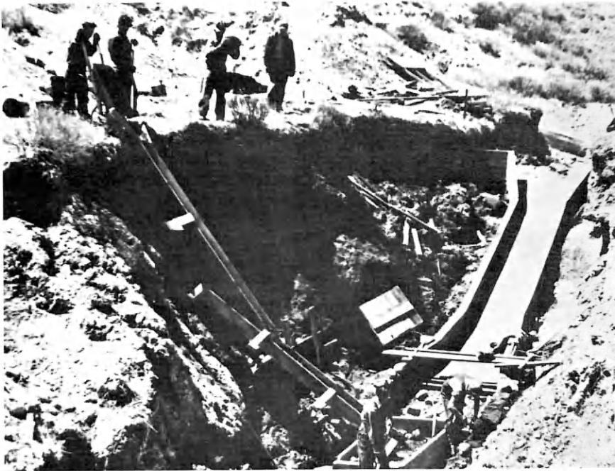
Lining of ditches to prevent soil erosion at CPS #5
