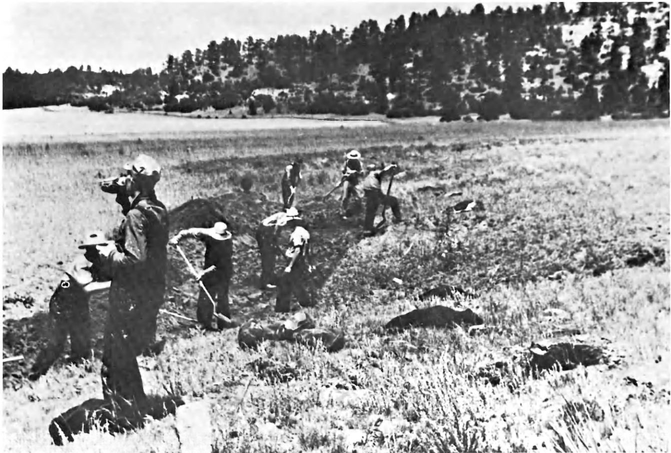
Diversion ditch construction at CPS #5
