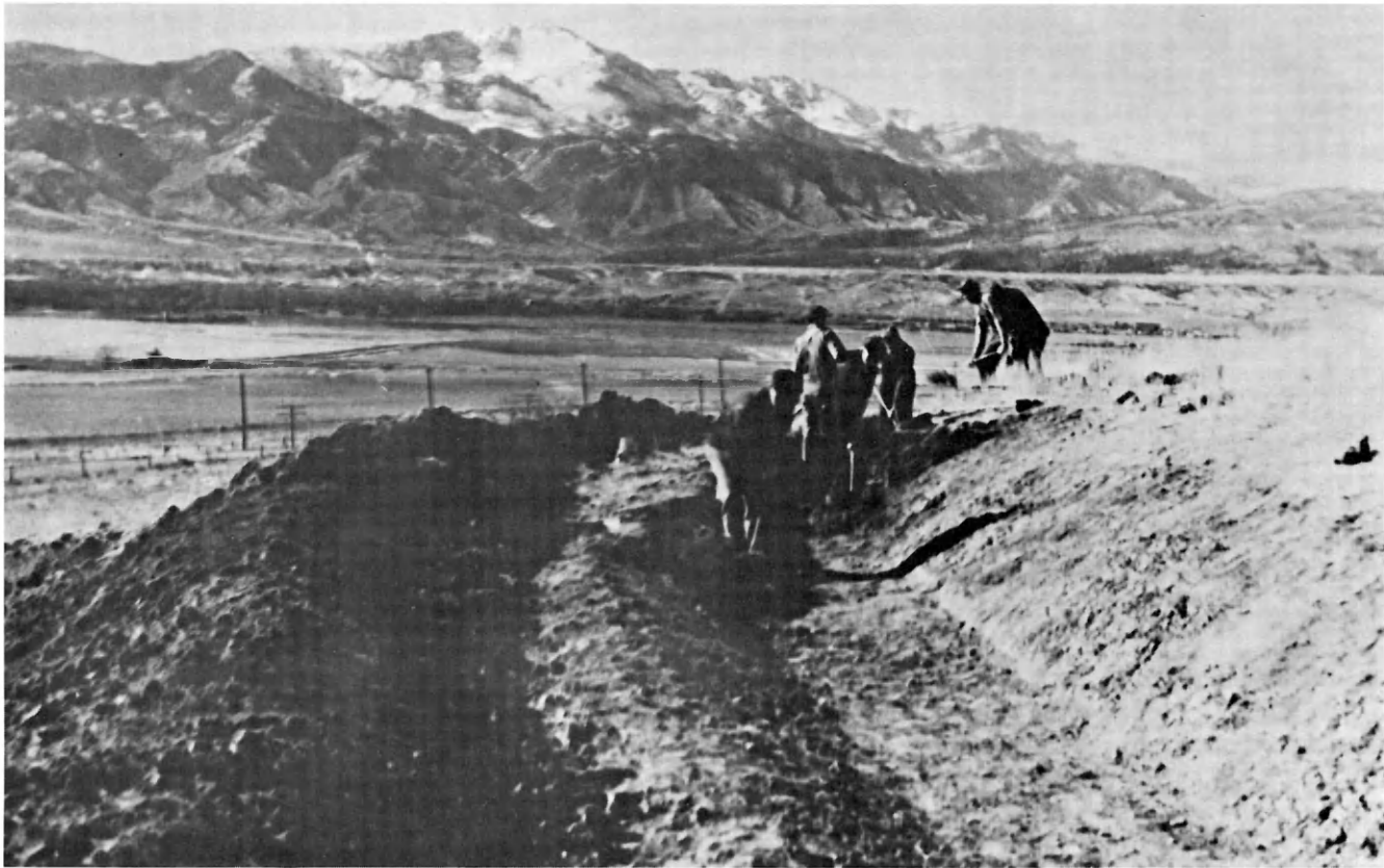
Diversion ditch construction at CPS #5
