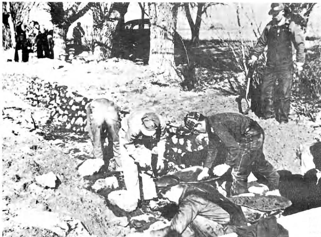
Lining irrigation ditches with stone and cement at CPS #5
