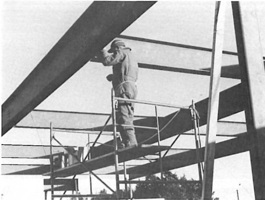
Construction manager Terry Doerksen works on steel beams. Photo: Larry Goering.
