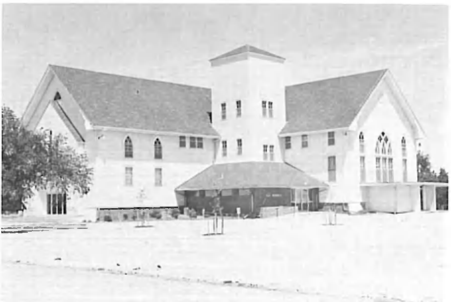
Top. This Eden Church building was dedicated in 1924. Four carpenters oversaw the volunteer workers who built it in less than a year. Men used the west (left) entrance, women the east. Middle. A 1949 remodeling project extended the building on three sides. An east balcony was made into classrooms. Bottom. In the 1950s an east entrance was added (right), putting in stairs to the children's classrooms in the basement. In 1982 an elevator for the handicapped, additional restrooms, and a brick entrance were built (center). Photos: Delbert Goering.
