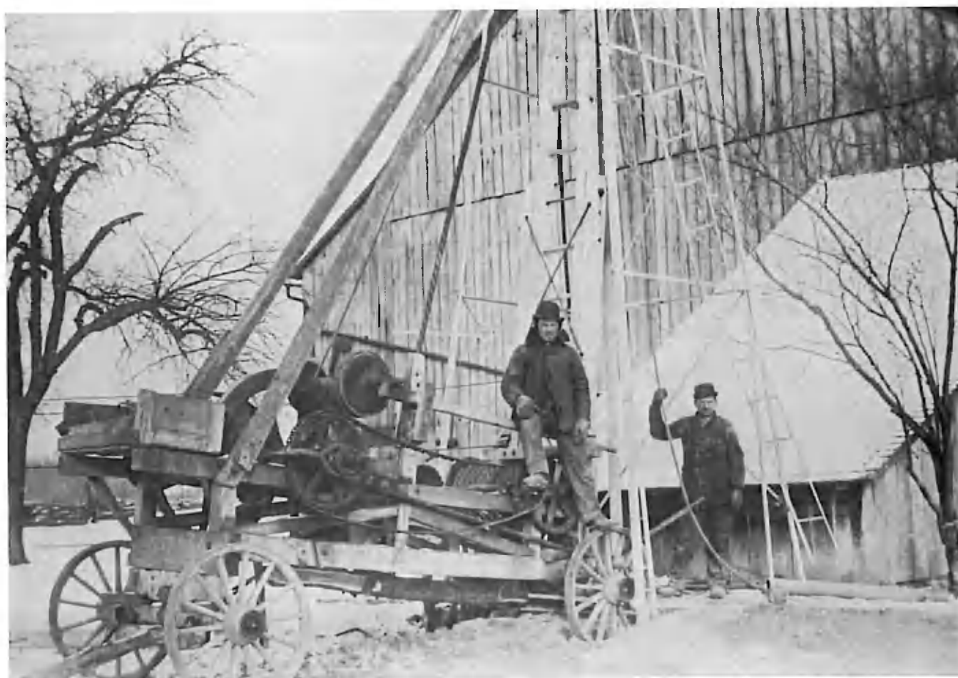
Right, Berry Brothers steam-operated well drilling machine; below, Pete Baumgartner's drilling machine.
