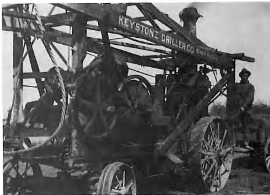
Right, Berry Brothers steam-operated well drilling machine; below, Pete Baumgartner's drilling machine.
