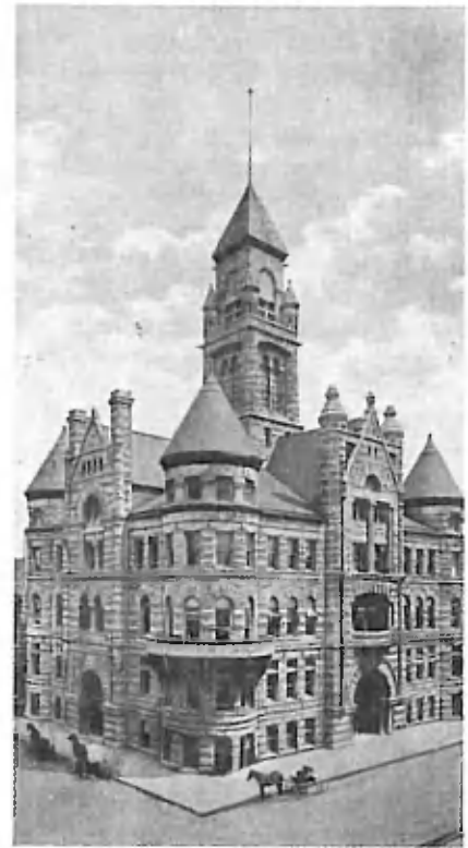
(Above) Wichita City Hall (Below) Salt Lake City and County Building
