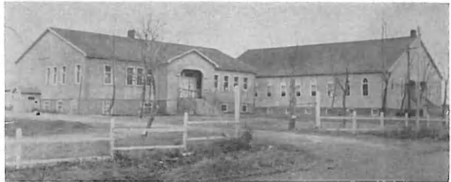
The Coaldale Mennonite Brethren Church built in 1934 with the enlarged Bible School building, above. Below, the old Coaldale hospital.
