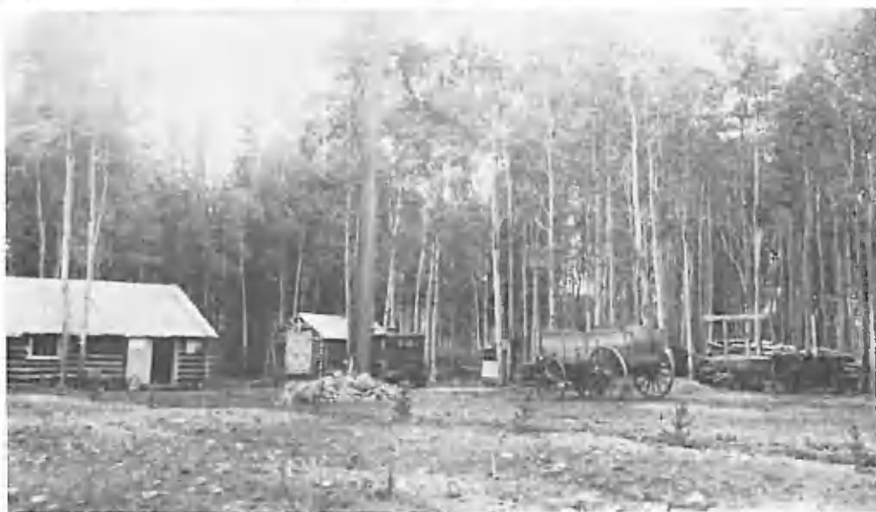
Cheslatta, B.C. August 15th, 1940. Buildings on farm of J. J. Martens on NW¼ of Lot 906. Granary in background is used as community storage house.
