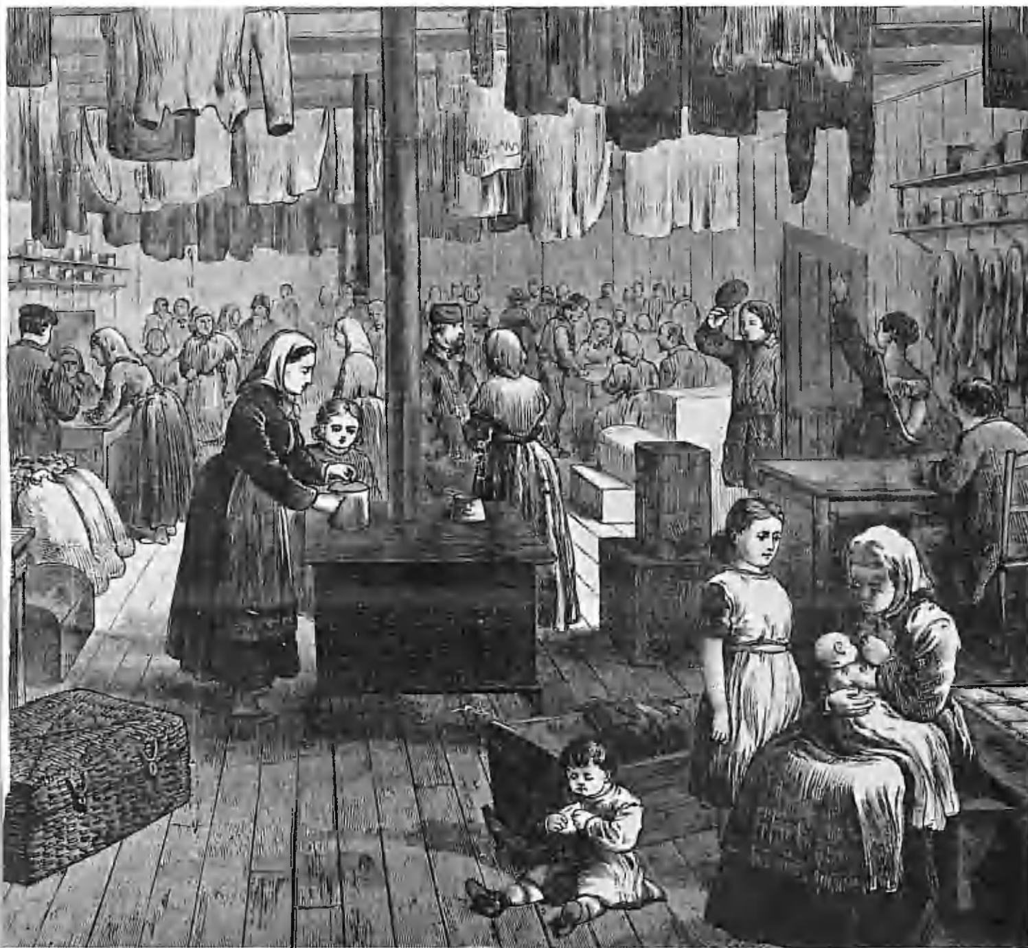
Interior view of one of the Mennonite immigrant houses in Kansas a century ago. The Santa Fe Railroad, from whom the Kansas settlers purchased their land, assisted in erecting five temporary houses of this type in various communities.
