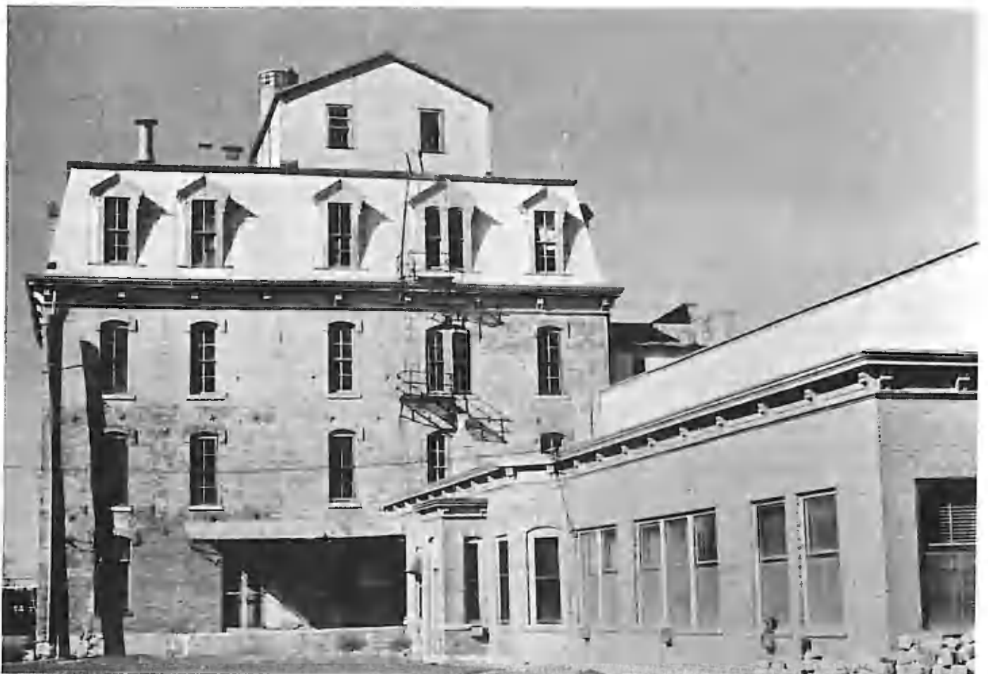
Below: East view of the Warkentin Mill in Newton as it appeared in early 1973, before restoration began. Originally built as the Monarch Steam Mills in 1879, the mill was bought and remodeled in 1886 by Bernhard Warkentin to handle the hard winter wheat which required different milling processes. (Photo by John F. Schmidt)
