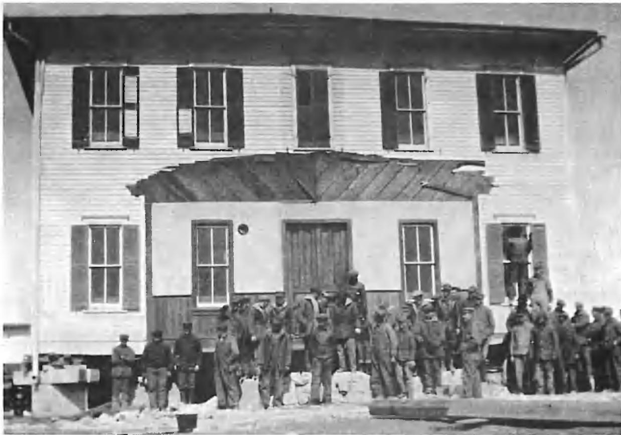
In early 1928, the wings of the Alexanderwohl Church were removed and the structure raised 39 inches in preparation for remodeling.
