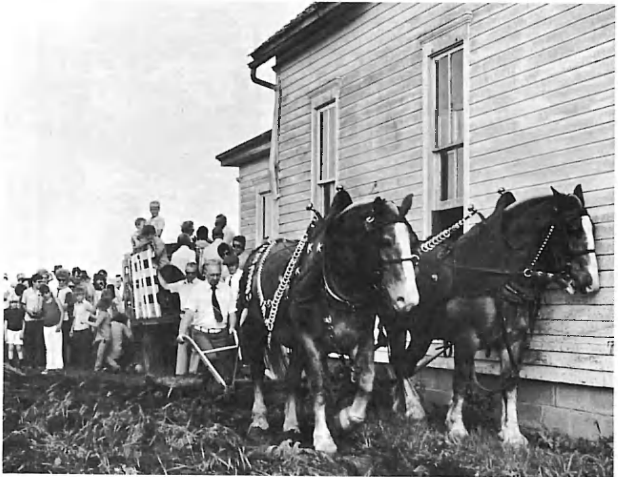
An old-fashioned walking plow was used to break ground for the museum complex now under construction at Goessel, Kan. Here Otto D. Unruh, a member of the foundation board, takes his turn in manning the plow. At the right is the building of the former Goessel Preparatory School, which was moved to the museum site.
