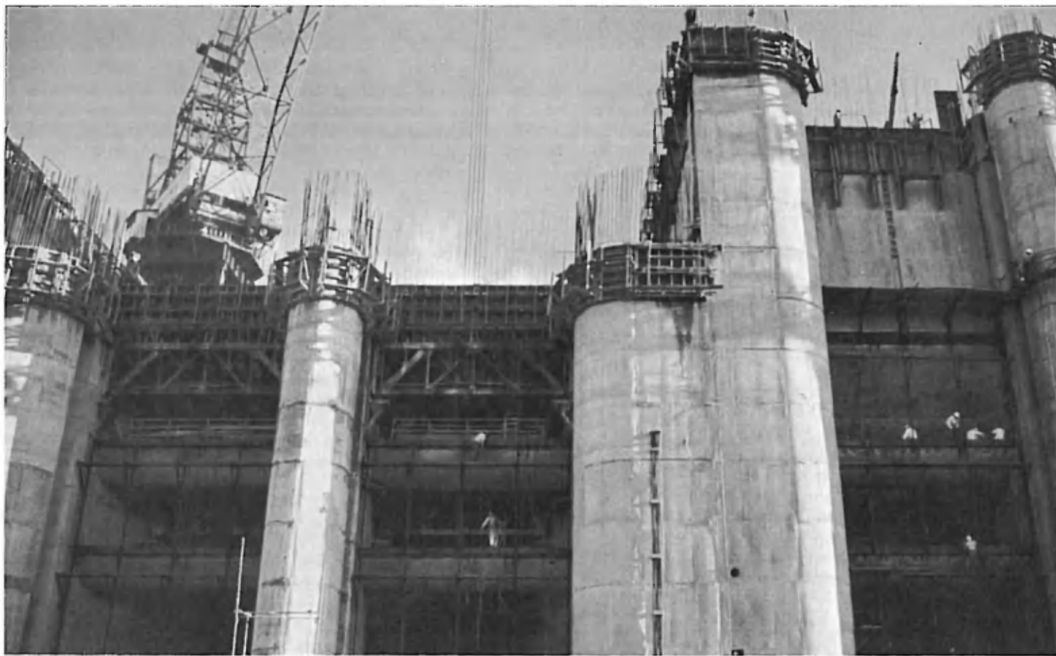
Generators at two new dams on the Parana River in southern Brazil will form one of the world's largest hydroelectric systems.
