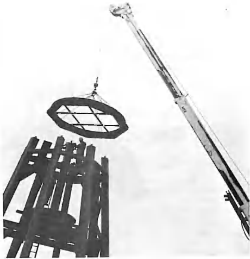
The ring is lifted into place. On top of this, the cap and fan-tail will revolve, directing the blades into the wind. Cost of the project was about $100,000, with the Manitoba government contributing $50,000
