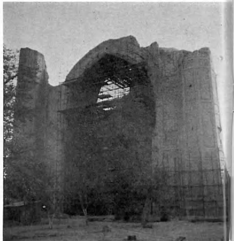
Mosque Bibi-Khanym in Samarkand under reconstruction.
