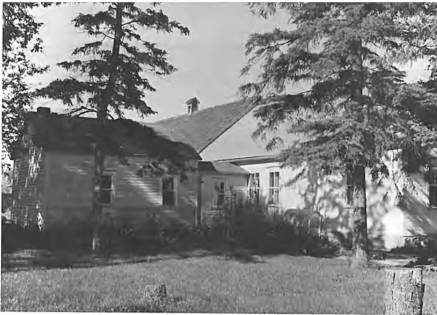
The summer kitchen is linked to the dwelling place.
