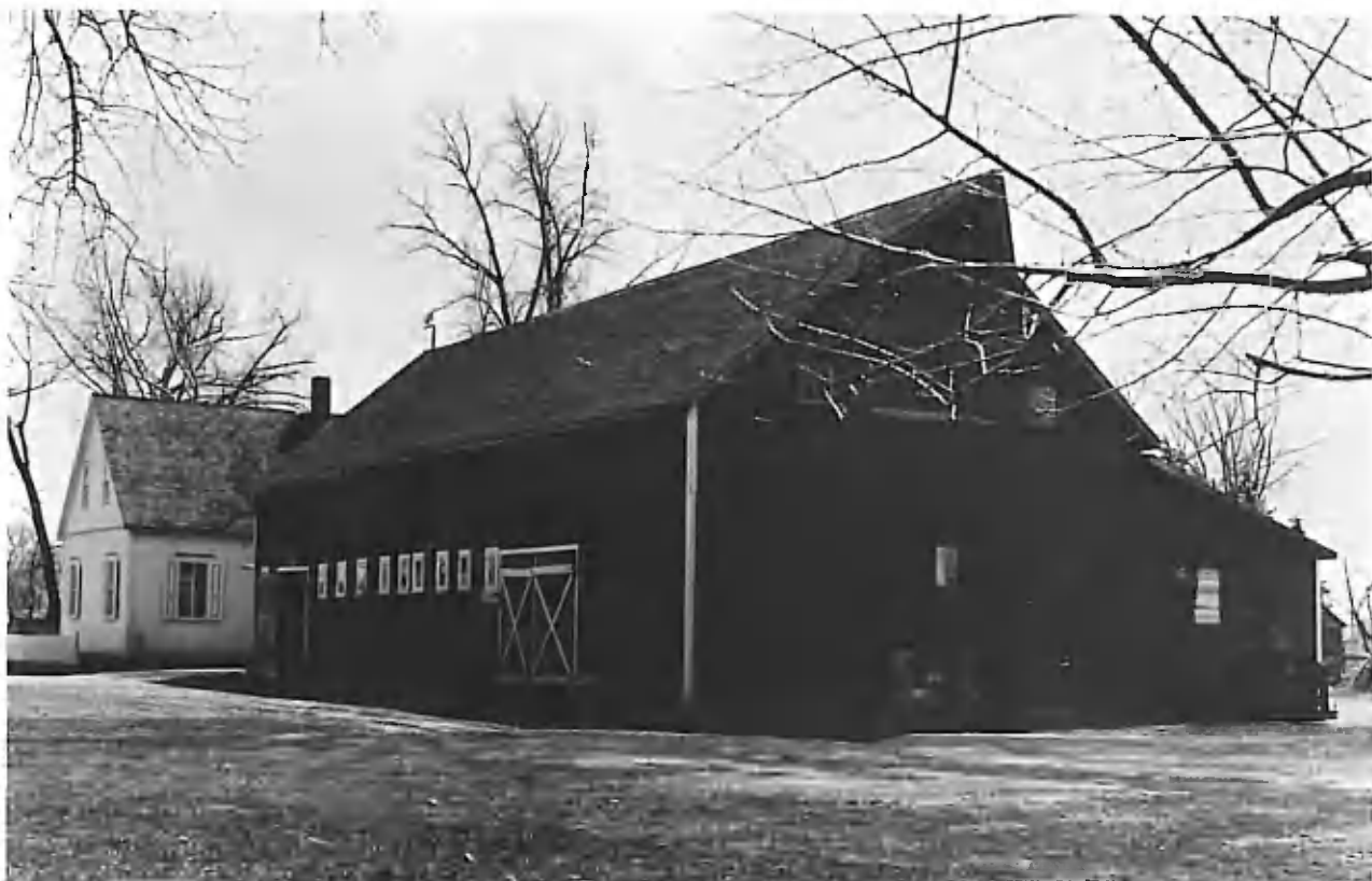
The traditional barn windows are enlarged and smaller in number.
