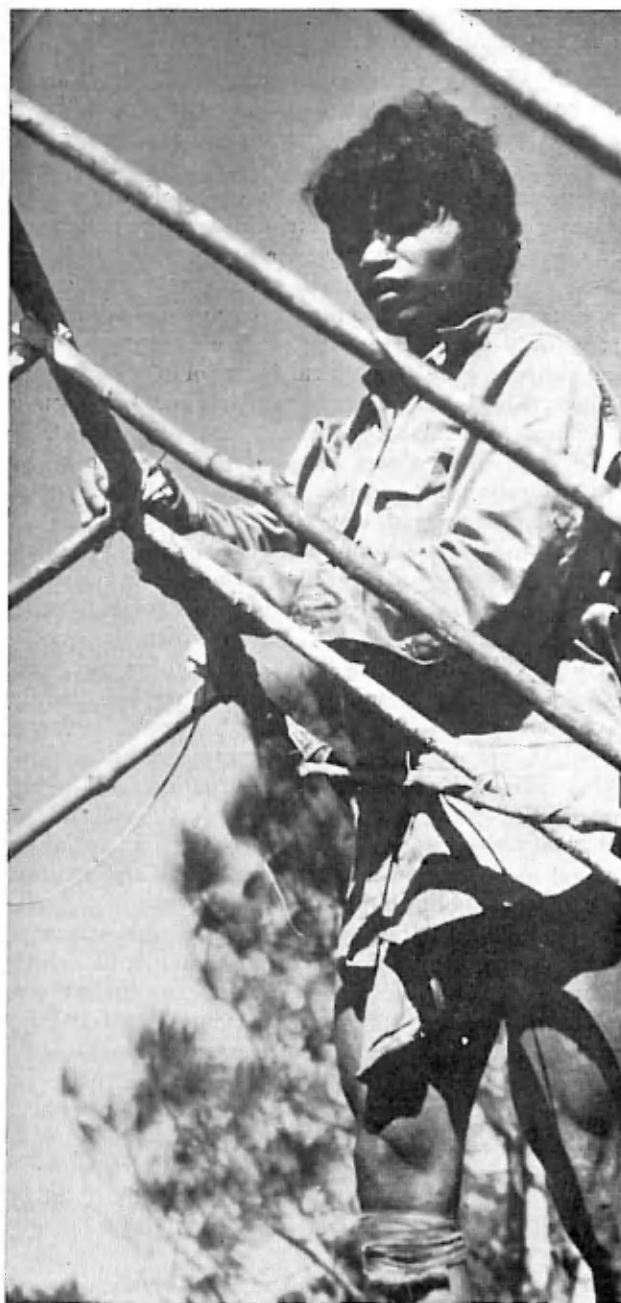
Roof construction by a Montagnard refugee.
