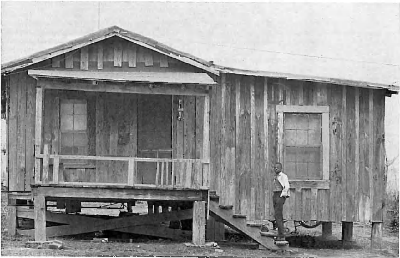
Typical house occupied by Negroes in rural Mississippi.
