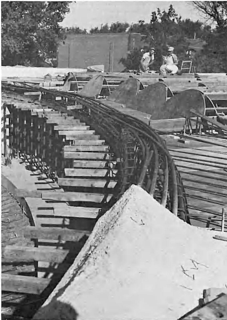
Steel rods circle the Fine Arts Center to support the dome-shaped roof.
