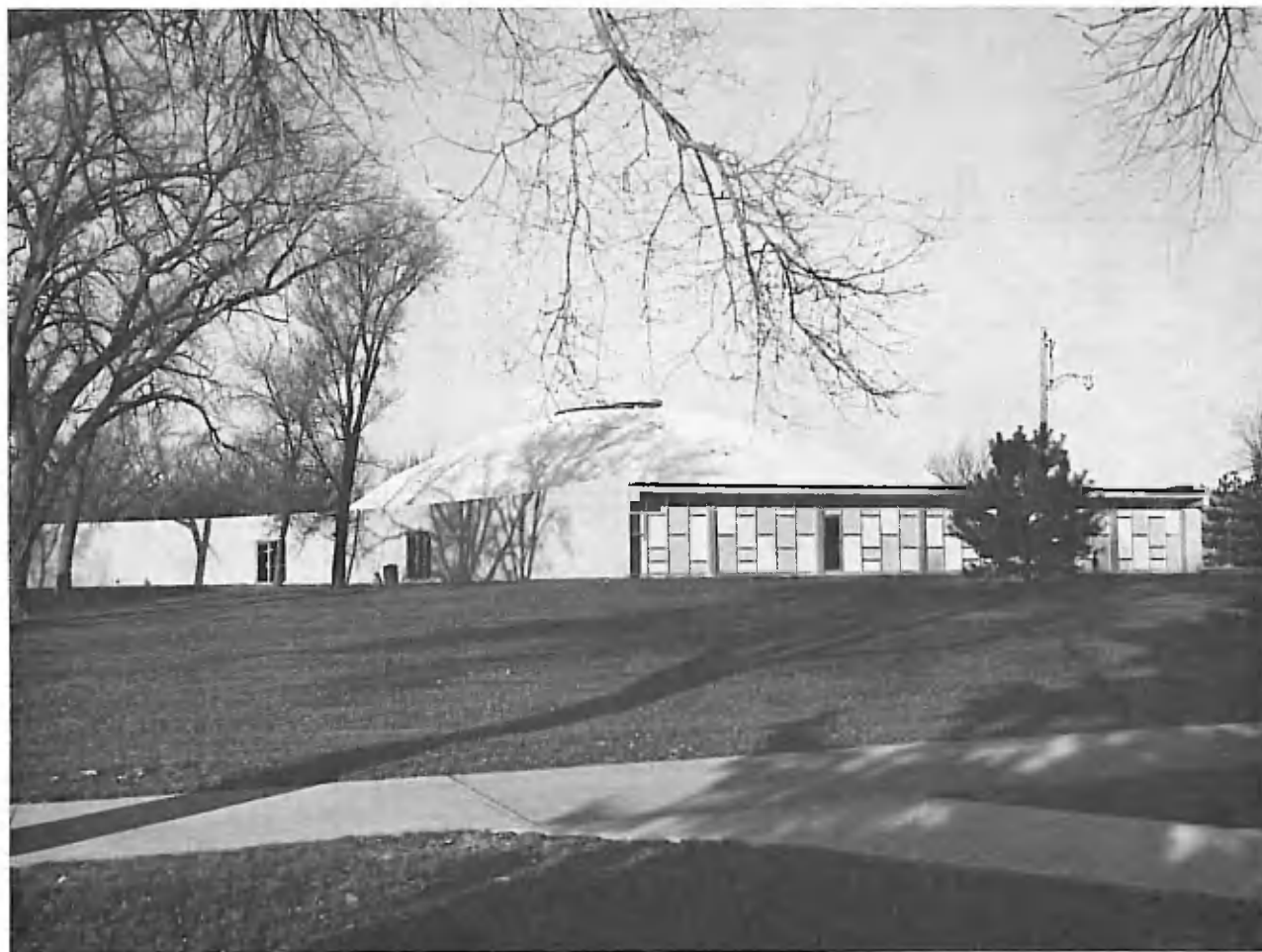
The east side of the completed Fine Arts Center.
