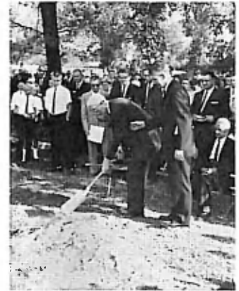
Ground breaking for Fine Arts Center at Bethel College in the fall of 1963. Participating David H. Richert, H. E. Suderman, and Vernon Neufeld, president.
