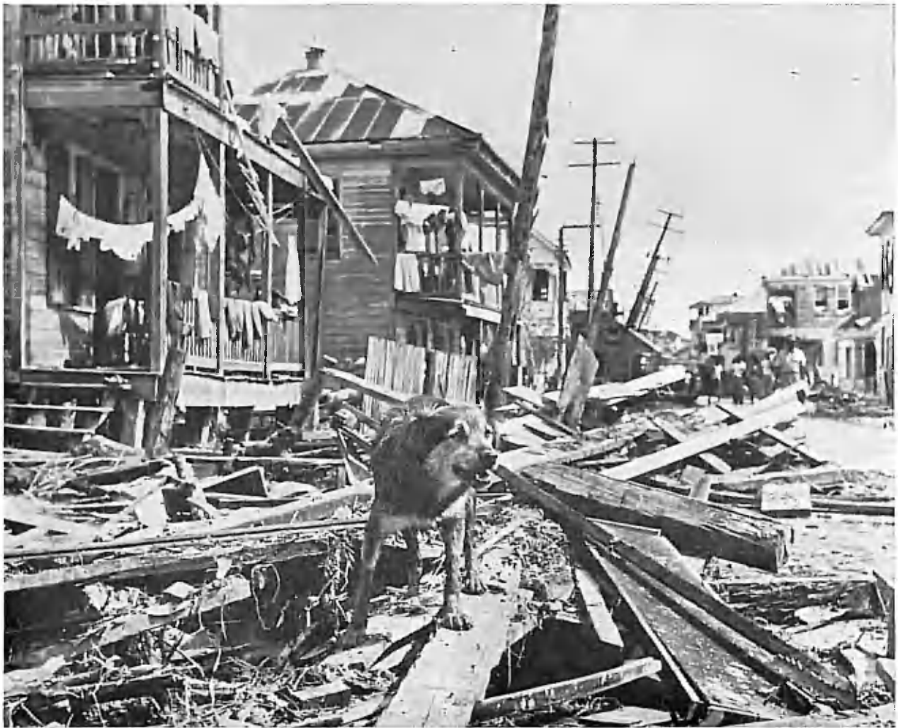
Dog guards remains of home at Belize, British Honduras after Hurricane Hattie had gone through.
