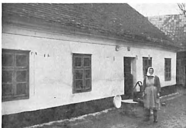
Former ceramic workshop of Hutterites now used as home located at Dehtze.
