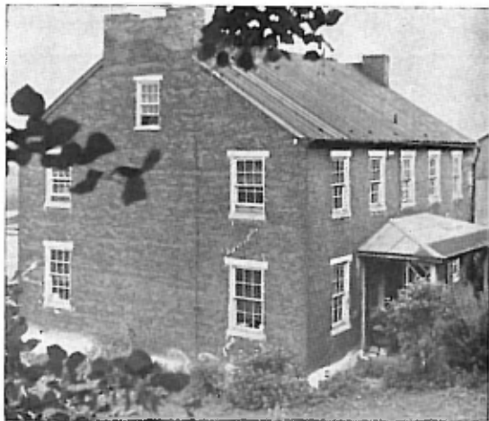
Farm building in Jacobs Creek Valley near Scottdale, Pennsylvania.
