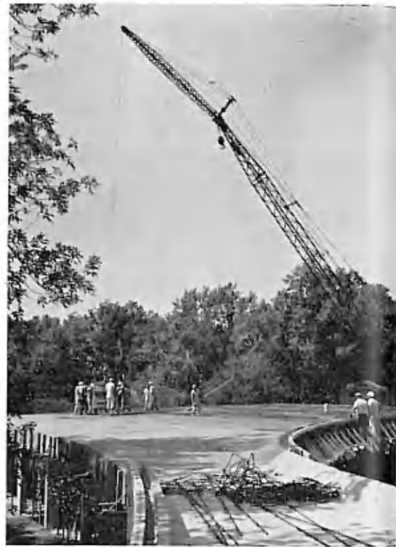
Construction of Bethel College Fine Arts Center.
