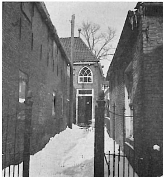
A hidden church in Poppingawier (Friesland)
