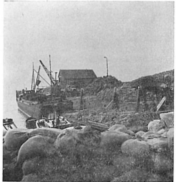
Supplies to repair flood damage
