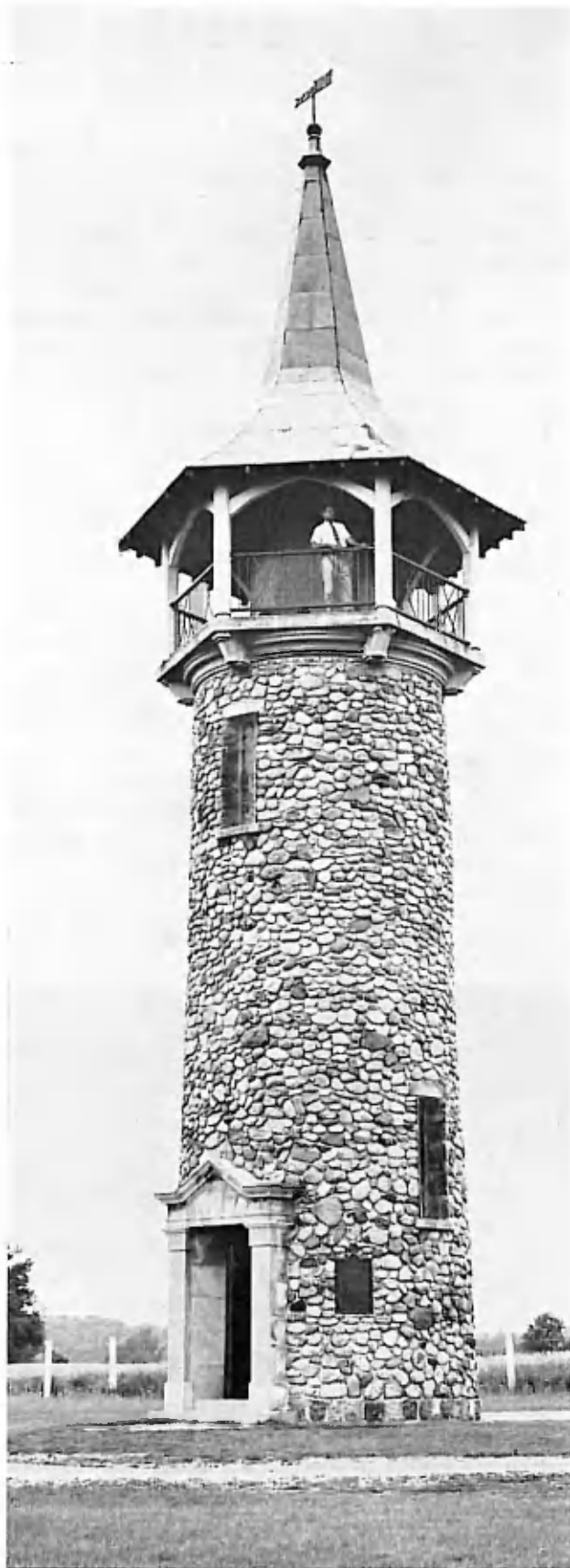
Old Pioneer Tower, Kitchener, Ontario.
