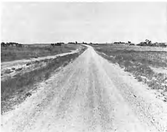
Completed roadway with crushed stone surface.
