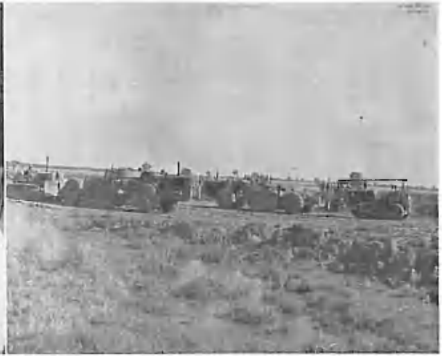
Scrapers and bulldozers working in the borrow pit.
