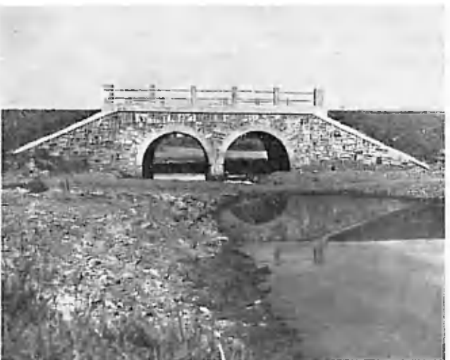
Double masonry arch culvert near Villa Hayes.
