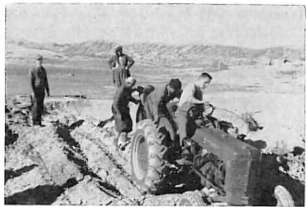
Breaking ground for administration building of demonstration unit.
