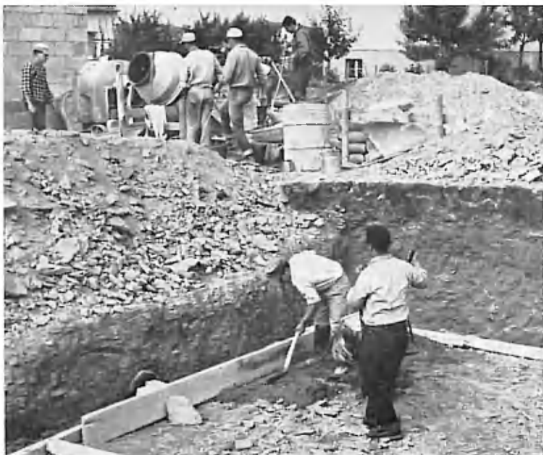
Pax crew begins pouring cement in hand-dug basement.
