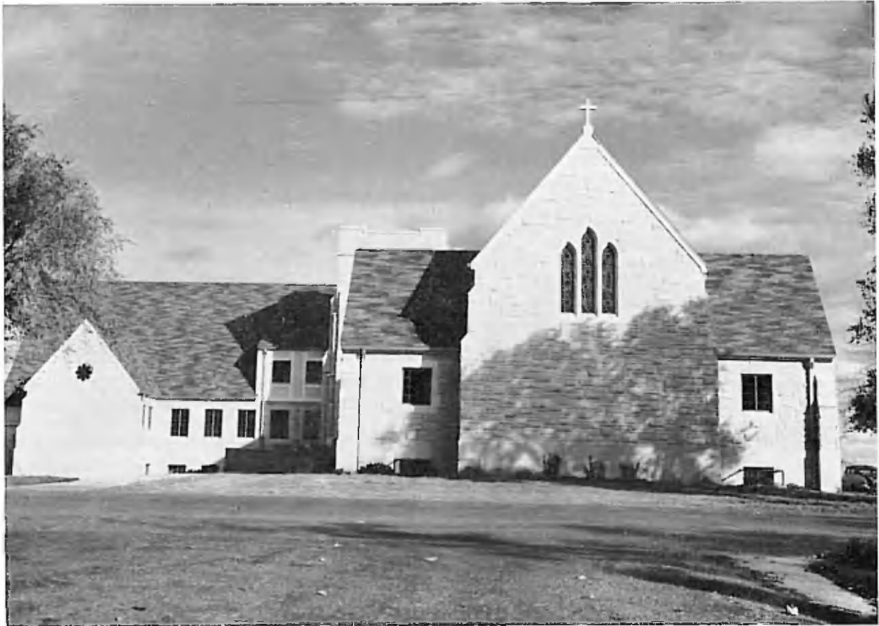
West view of Bethel College Mennonite Church, dedicated December 2, 1956
