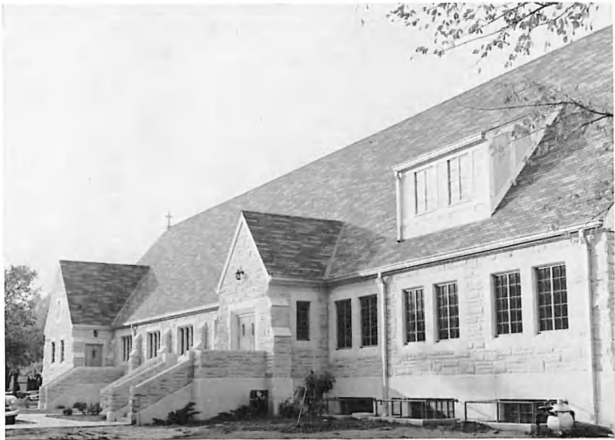
View from southeast showing south entrance to sanctuary. Hewn rock is native limestone.
