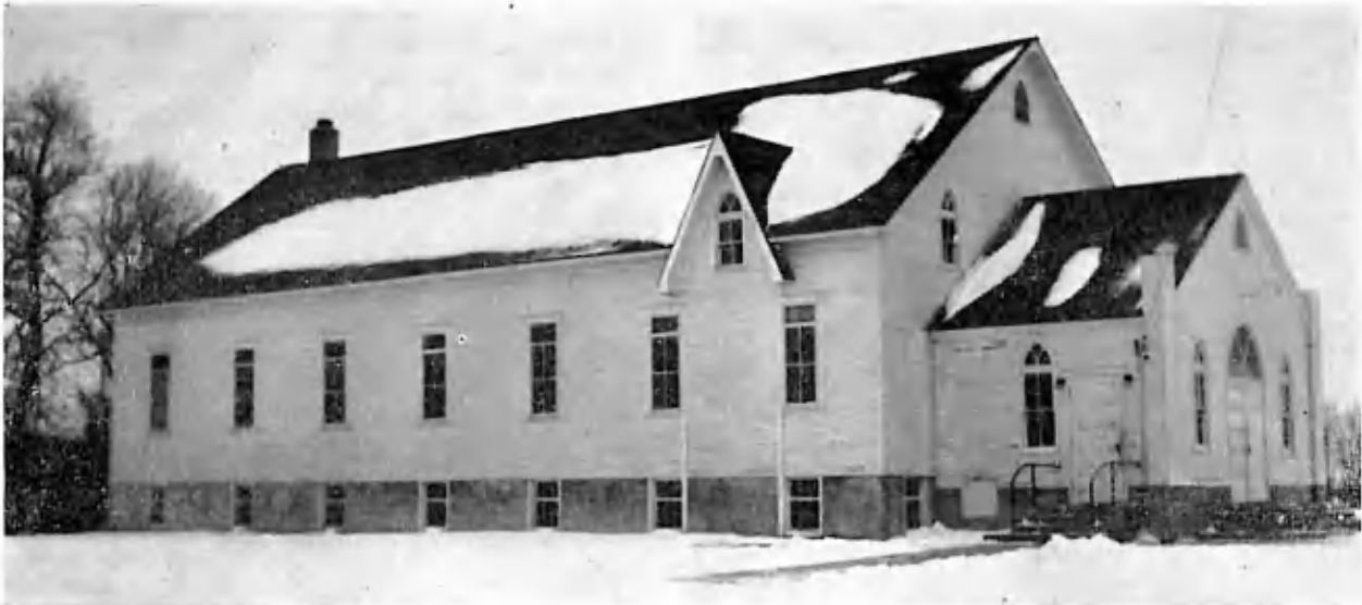
Old church building of the Kleine Gemeinde, now Evangelical Mennonite Brethren Church of Steinbach. Today its Sunday school enrollment numbers 400, the largest of any church in Steinbach. This church was enlarged some time ago. A new structure in the foreground is a much larger church now in construction. (Left, below) Bergthal Mennonite Church of Steinbach. (Right, below) Lutheran church whose membership consists of German descendants who settled in the district south of Steinbach in 1900. This is one of the two non-Mennonite churches of Steinbach.
