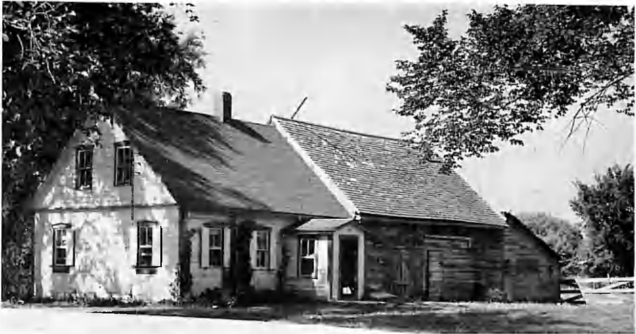
One of the original typical Mennonite homes still standing in the Steinbach district. The first part is the dwelling place joined directly by the barn. The ham curing chamber is usually located in the back yard. Some of the homes were more elaborate.
