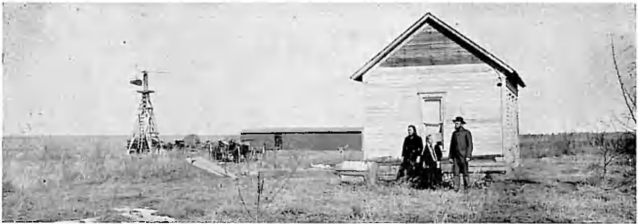
Homestead of Isaac Regier, north of Enid, Oklahoma, 1894. (Below) Plowing with the Iron Horse, 1907.
