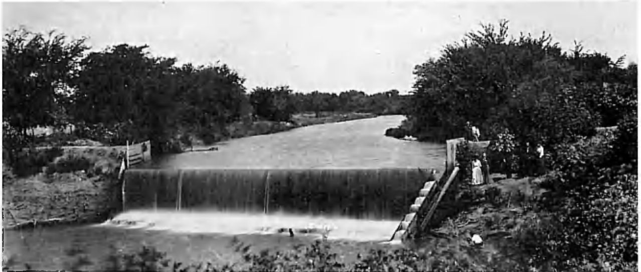
The Alta Mill dam, established in 1878, had a 23-inch water turbine. In 1885 a new dam was established which was washed away in 1918.
