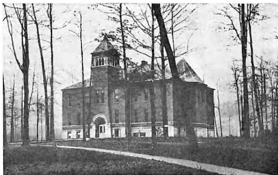
College Hall, built 1900.
