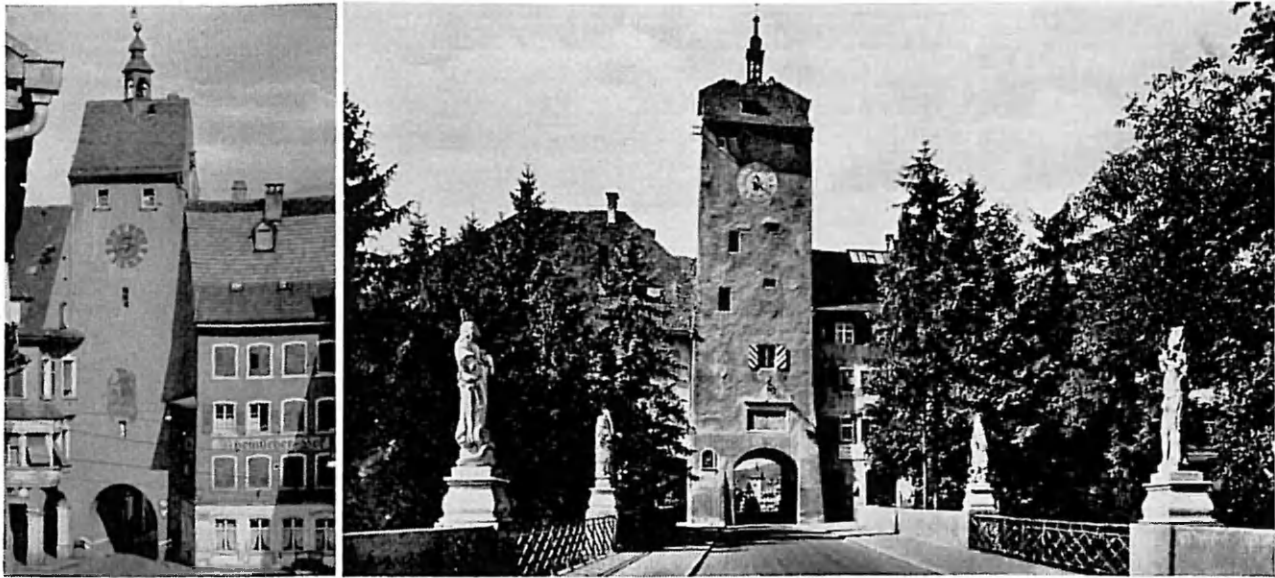
The lower gate and the upper gate of the old city of Waldshut along the Rhine in South Germany.
