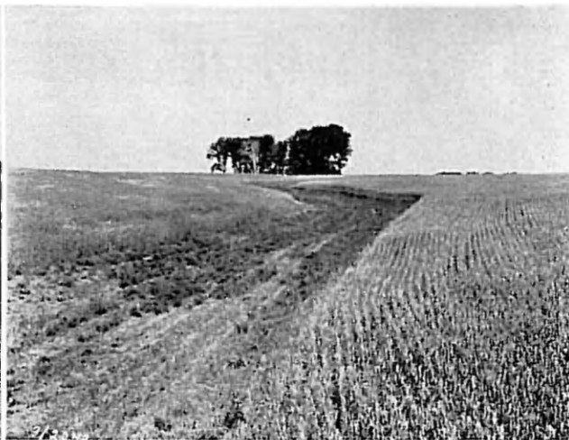
Shaped and seeded drainage ditch in North Dakota and same ditch with stand of brome grass and alfalfa.
