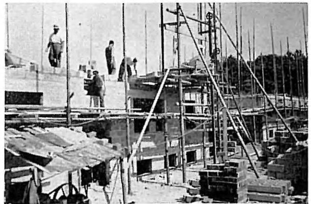
Making building blocks from lava deposits and cement. Third and fourth houses in Backnang going up.
