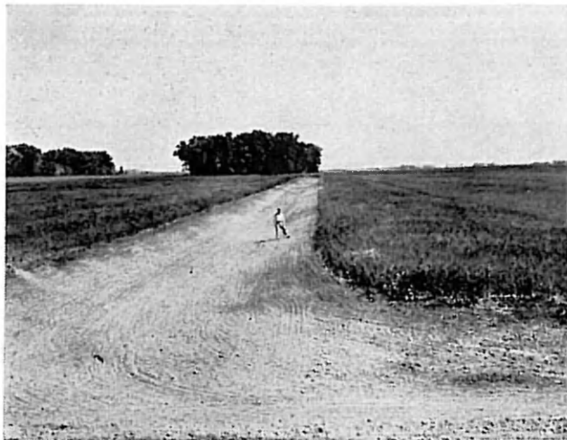
Shaped and seeded drainage ditch in North Dakota and same ditch with stand of brome grass and alfalfa.
