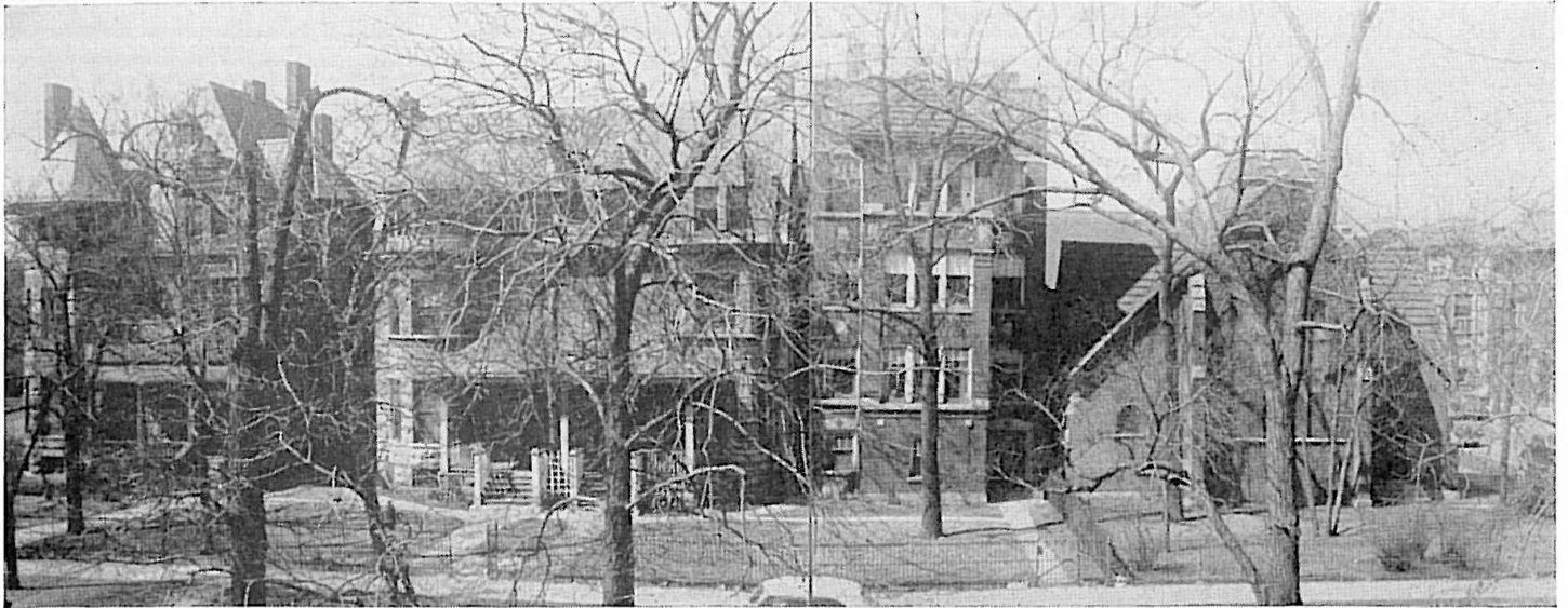
Mennonite Biblical Seminary buildings on Woodlawn Avenue showing Main building, Franz Hall, Memorial building and Woodlawn church.
