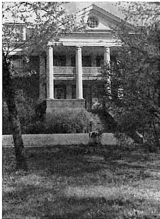
Ropp Hall, Bluffton College dormitory and dining hall.
