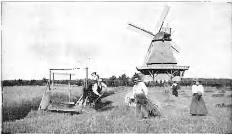
With McCormick's reaper a two-man crew could cut as much grain as four or five men with cradles.
