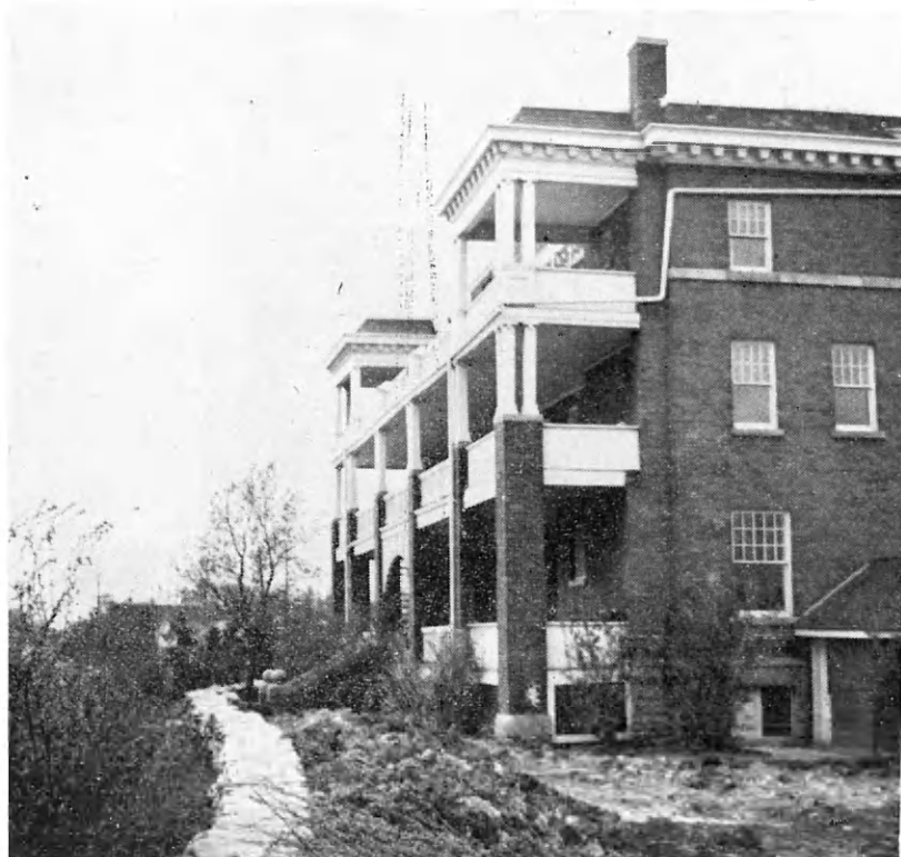
Concordia, a 50-bed hospital near Winnipeg.
