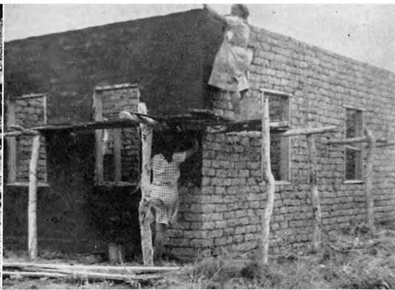
(Top) Their husbands and brothers in Siberia, these women are building their own homes with adobe brick in the Chaco. (Left, top and center) Meals are being prepared and served under primitive conditions.
