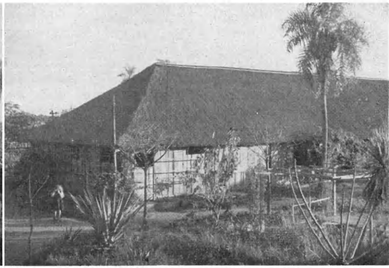
(Top, left) Lumbermill and workshops. (Top) One of first buildings, still being used. (Left, center) Interior of dining room on the "Loma Jhoby." (Left, bottom) Sowing on the fields cultivated by the Hutterite brethren.
