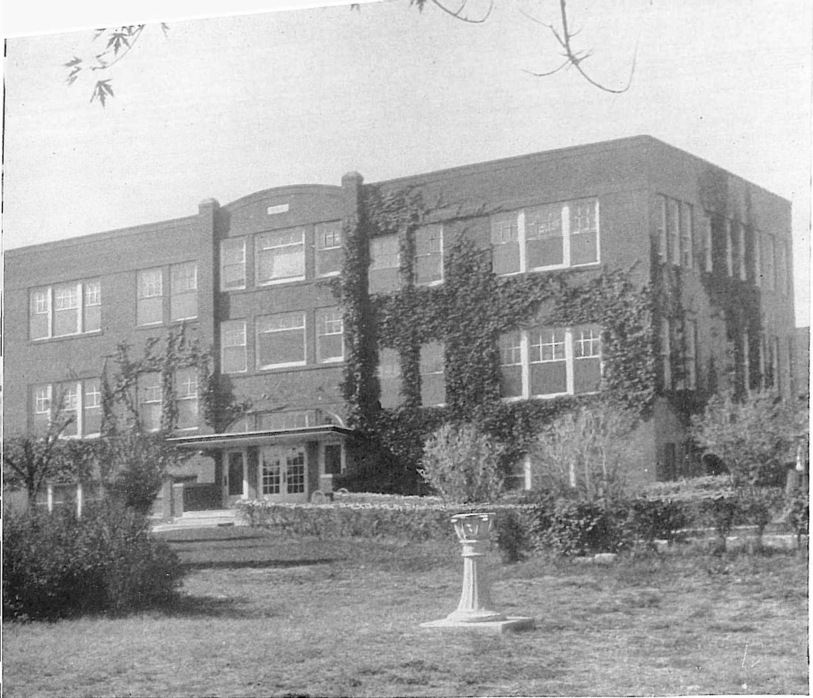
Administration Building, Hesston College, in use for thirty years for offices, classrooms, and assembly hall.
