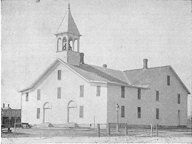
The former Berne Mennonite church, replaced in 1912.
