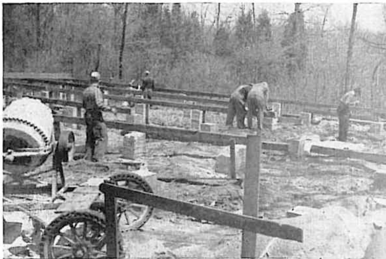
Building an auditorium.
