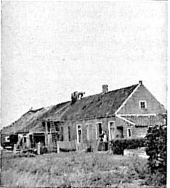
MCC unit repairs a damaged house on Walcheren Island (Holland).
