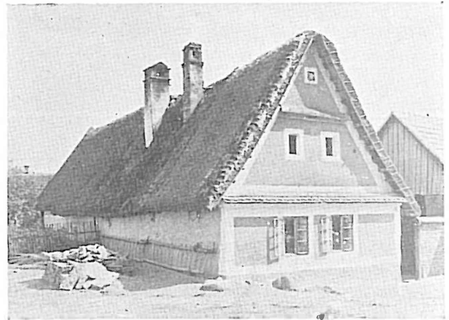
Habaner building in Sobotiste
