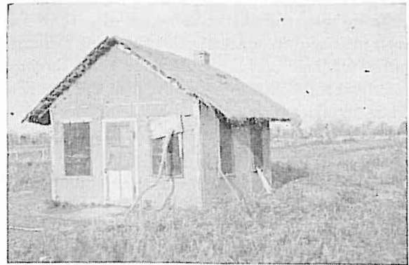
4. One of the earliest school houses in Menno Colony, very thin walls of adobe clay, grass roof, no glass in the windows, only black shutters. Still in use in 1939.
