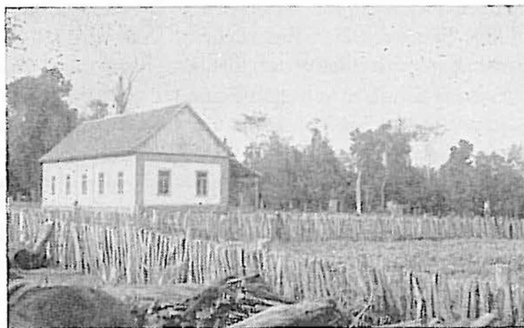
5. A beautiful 1945 two-room school house in Friesland Colony, walls of substantial adobe clay painted white, rooms well lighted, equipped with glass window panes. Playground ample and well-kept.
