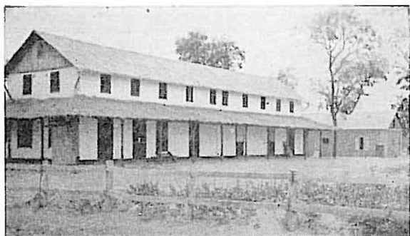
7. Hospital building in 1939. Doctor's office at near end, patients' quarters at the other, nurses' quarters second floor, unbearably hot in high temperatures. Wide veranda protects walls from rain and rooms from excessive heat.
